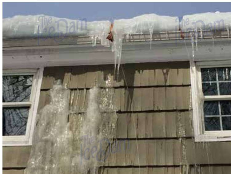
These salt socks didn't melt down to the roof, resulting in massive water damage to the interior walls. (Can you find the ice on the siding?)
