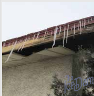
SOFFIT DAMAGE
