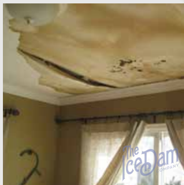
WATER DAMAGE
