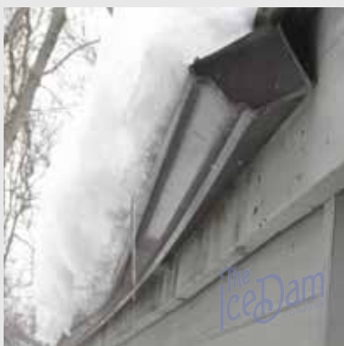
GUTTER DAMAGE
